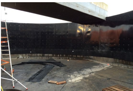
PE-HD vlakke renovatiebeplating
