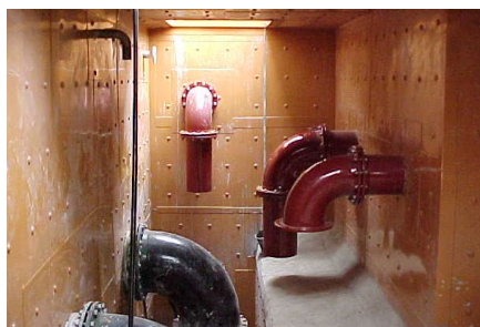
PVC vlakke renovatiebeplating
